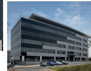
CFC Admin Building tinted Euro Grey
